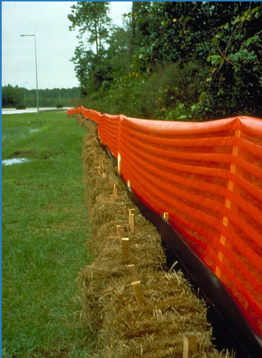
Plate 4.05b Construction of a Straw Bale Barrier Source: NRCS
